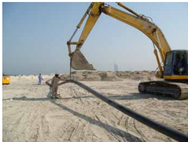
Pipe handling during the pullback operation.
